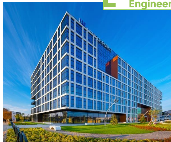
Project: AFI Tech Park Surface: 1,250 sqm
