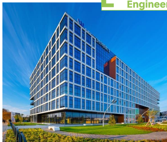
Project: AFI Tech Park Surface: 1,250 sqm
